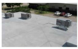
Another factor in replacing the roof of a television station facility is the number and scope of penetrations for antennas and satellite dishes—a detailing nightmare for conventional roofing systems. As a spray-applied system, polyurethane foam makes detailing easier, providing leak-free protection at a lower labor cost.
