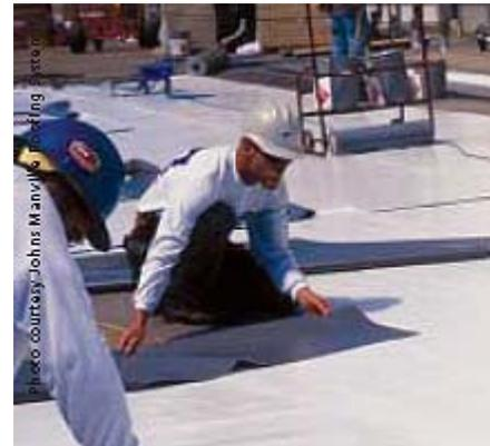
The performance properties of rigid-foam expanded polystyrene insulation generally reduce labor and material needs. EPS can also help provide an environmentally sustainable structure with long-term thermal resistance. EPS is custom-manufactured to meet specifications for the required R-value, compressive load, and other project demands that can help minimize waste.
